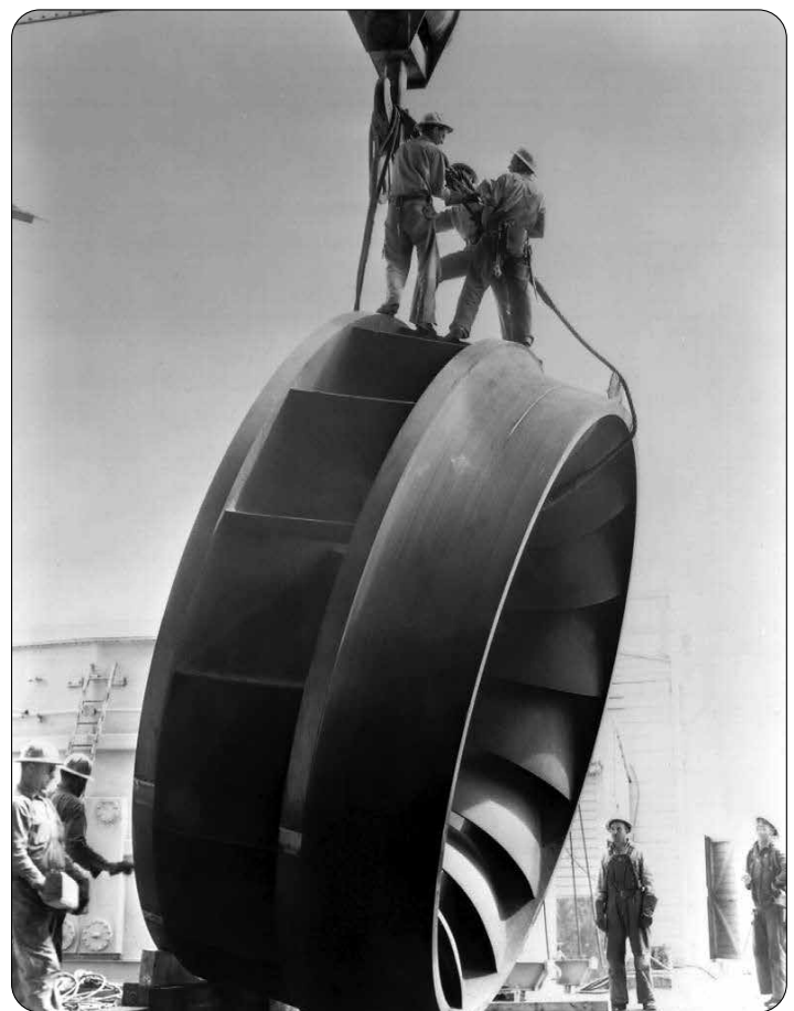
Workers install a Francis turbine at Grand Coulee Dam, 1947.
