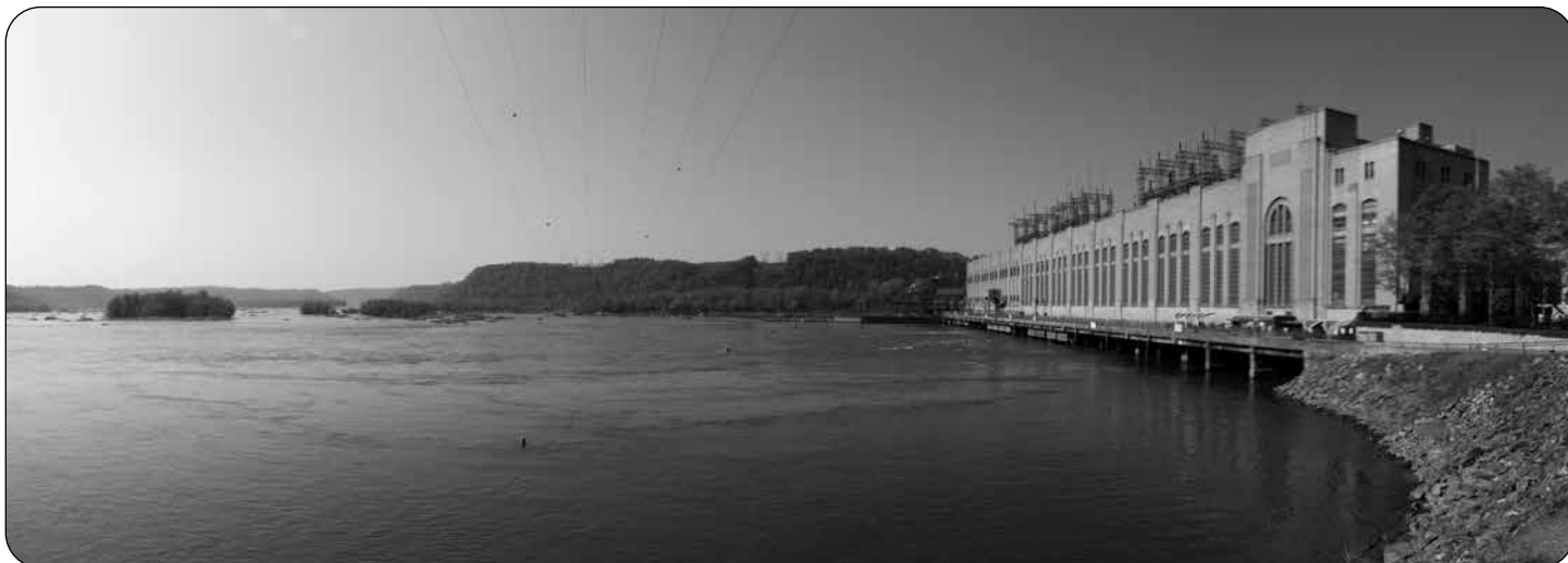
The down river side of a hydropower plant on the Susquehanna River in southern Pennsylvania.
