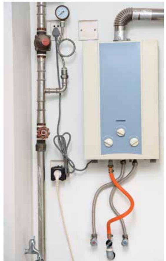
A continuous flow water heater only prepares hot water when it is needed.
